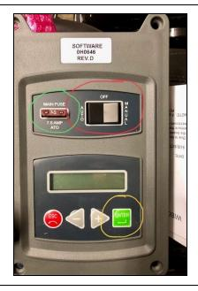
**STEP 3:** Put generator into "MANUAL" position on the controller. The generator will either start or make three (3) attempts at starting. If it starts, let it run 5 minutes, then put it into the "OFF" position.
