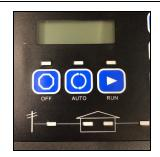
**STEP 3:** Push the blue "AUTO" button on the controller which puts the generator in AUTOMATIC/STANDBY position.
