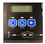
**STEP 3:** Push the blue **"RUN"** button on the controller. The generator will either start or make three (3) attempts at starting. If it starts, let it run 5 minutes, then push the blue **"OFF"** button.
